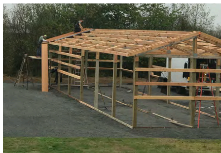
Garden Spring 2021 – New pole barn during construction.
