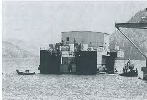
Picture: A large-floating fish collection facility is being positioned into place within the Swift Reservoir on the Lewis River, WA. (Picture taken by Bill Wagner from the Daily News, Longview, WA)
